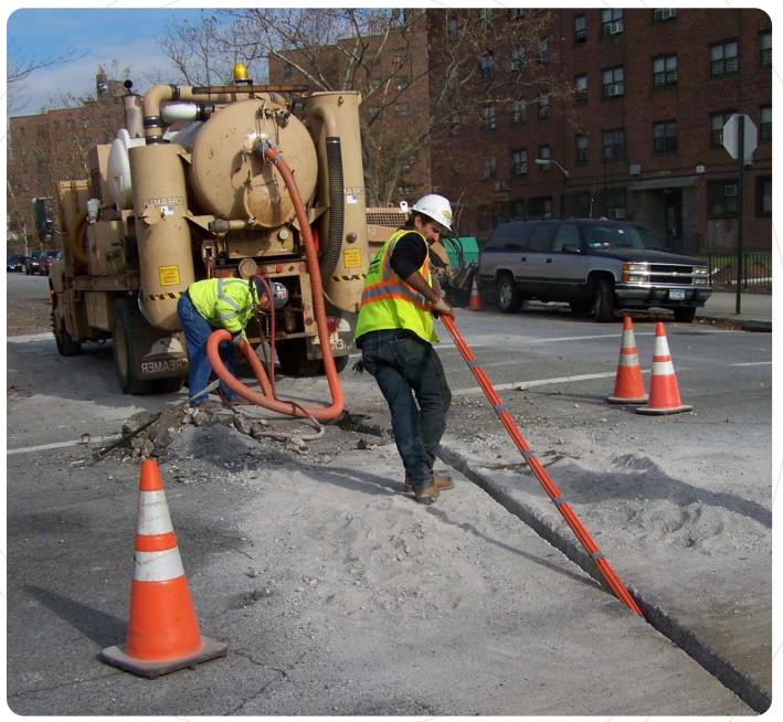
photos on opposite page top: FuturePath Flex 6-way install middle: FuturePath Flex transition from MicroTrench to underground bottom: With MicroTrenching there are no road closures; cars can drive over the open trench during installation.
